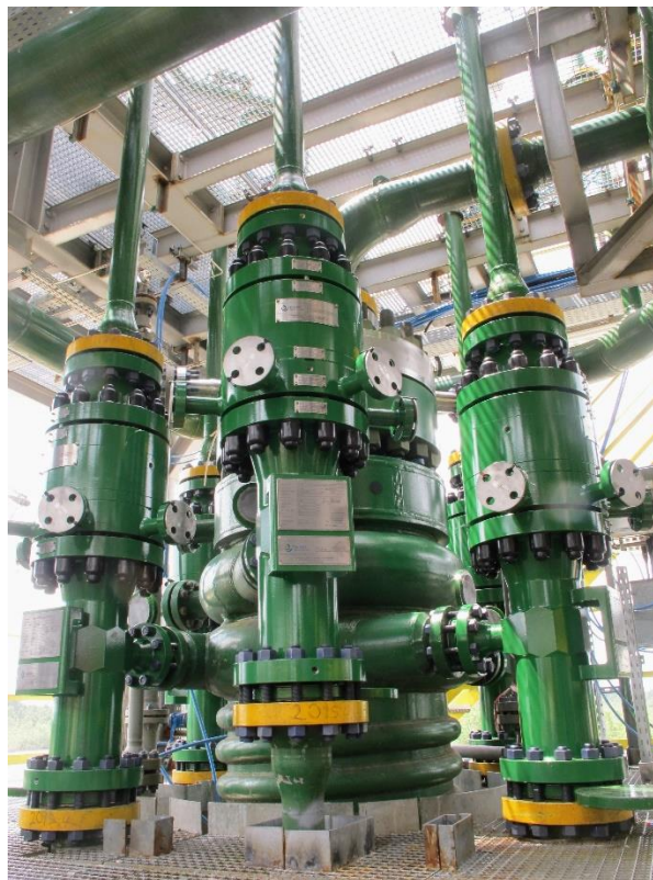
Figure 4: Up to 8 Twister Supersonic Separators can be connected to the Twister Hydrate Separator
